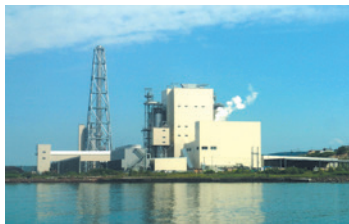
Mombetsu Biomass Power Plant
