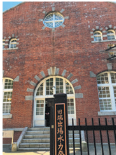
Hadeba Hydroelectric Power Plant
