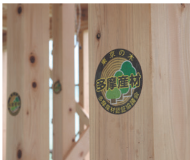
Japanese cypress from the Tama area used for pillars and foundations
