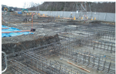
Pouring concrete for the foundations in bitterly cold weather
