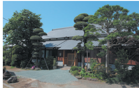
House exterior with retiled roof
