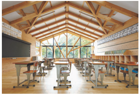
Extensive use of wood in a large open space with posts arranged in a tree-like structure
