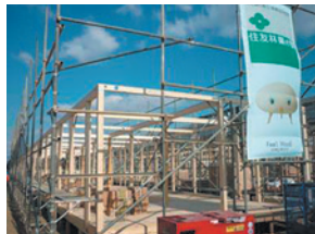
Erecting the frame
