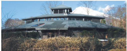
Exterior of the Forest Ark. Its design concept emphasizes harmony with nature. When viewed from above, the building resembles the shape of a leaf.
