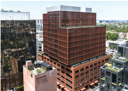
Jointly developed 15-story office building constructed with a mixture of wood and reinforced concrete
