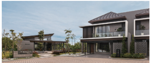
Spec home community project (Bekasi, Indonesia)
