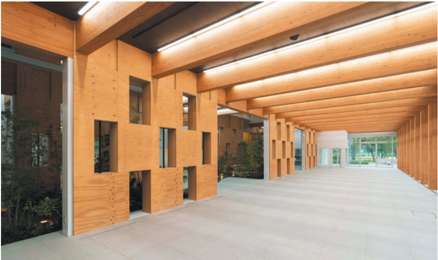
NPIL's LVL was used in the new research building at the Tsukuba Research Institute.
