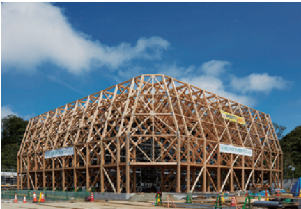
Structural framework of an indoor sports hall, Miyanomori Elementary School, Higashimatsushima City
