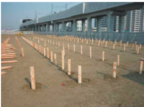
Wooden piling work
