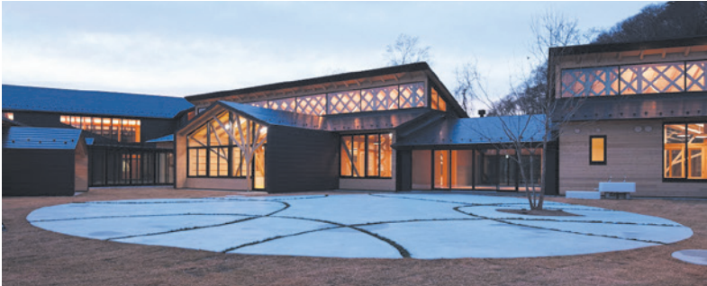
Buildings surrounding an inner garden and linked by connecting corridors
